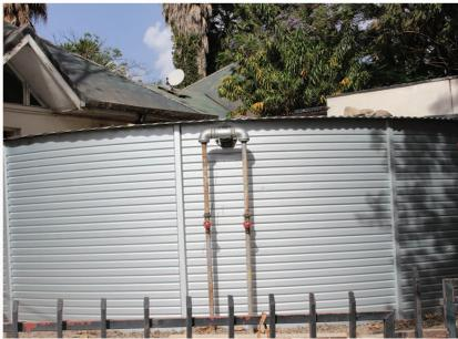
The Pioneer water reservoir, which is a reliable source of clean water should municipal pipes run dry, is designed considering into account all environmental conditions such as wind, seismic, static and sloshing loads.
